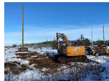
Installation of bog mat for transmission line 55L.
